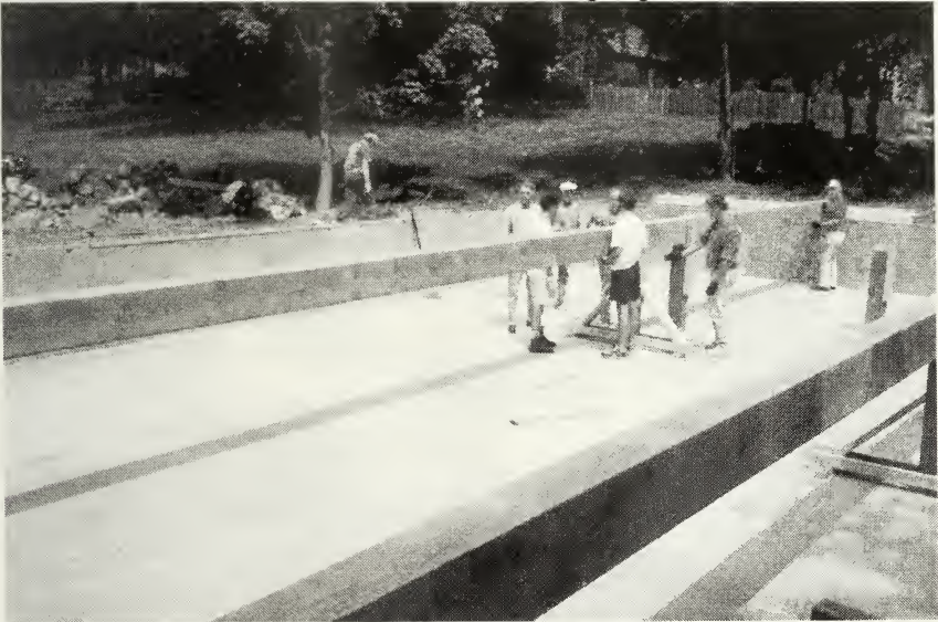
Massive floor joists installed by volunteers
